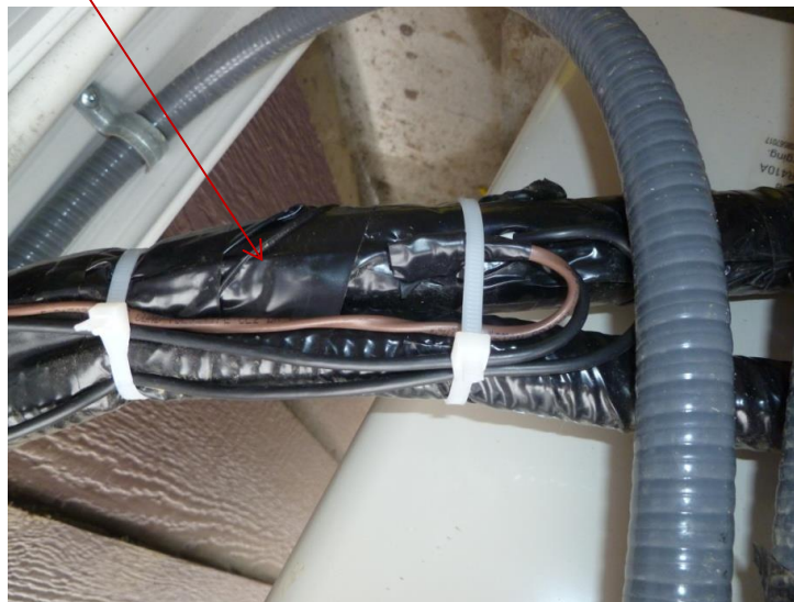
Figure 9. Vapor Line Thermistor
