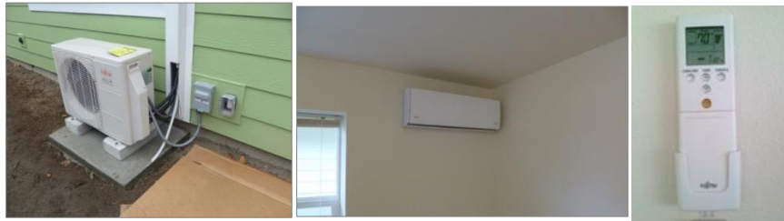
Figure 4. DHP: Outdoor, Indoor units and remote thermostat in living room
