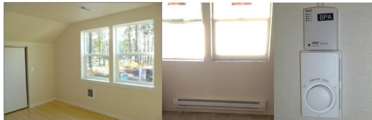
Figure 5. Electric Resistance, fan and baseboard types and hard wired thermostat in living room w/T/RH data logger
